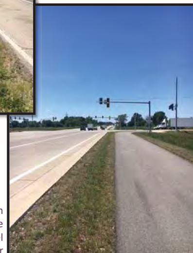
Example Bike Path with Minimum Separation and Bike Friendly Shoulder between Travel Lane and Curb and Gutter
